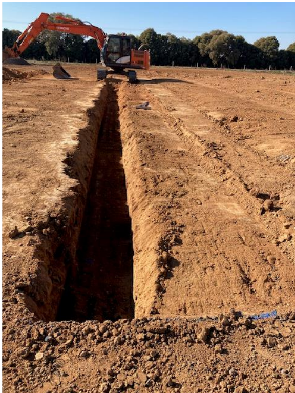
Image 16: Excavation for a Wick Trench
