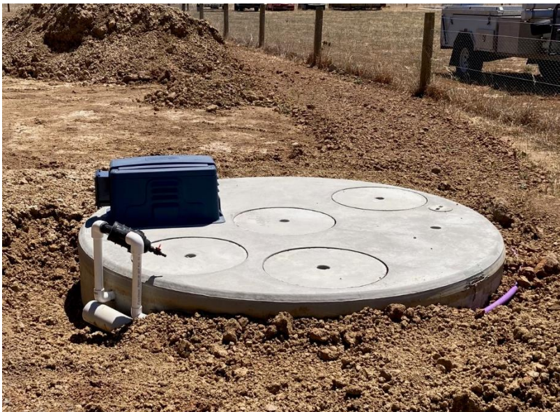
Image 9: Top of a packaged treatment plant – only the lid, control box and filter visible once backfilled
