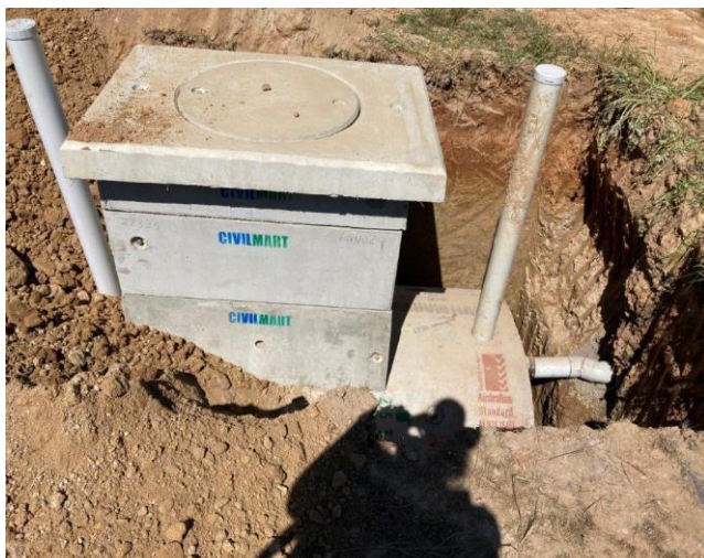
Image 7 – Septic tank with riser lids finished at ground level. All waste septic tank with risers extended to ground level to ensure access for pump out and other maintenance. Pump well installed at the outlet of the septic tank to pump to effluent disposal trenches.
