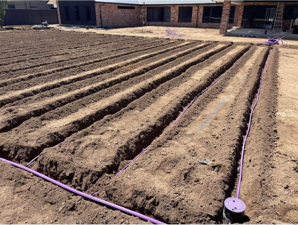
Image 18: pressurized sub-surface drip irrigation
