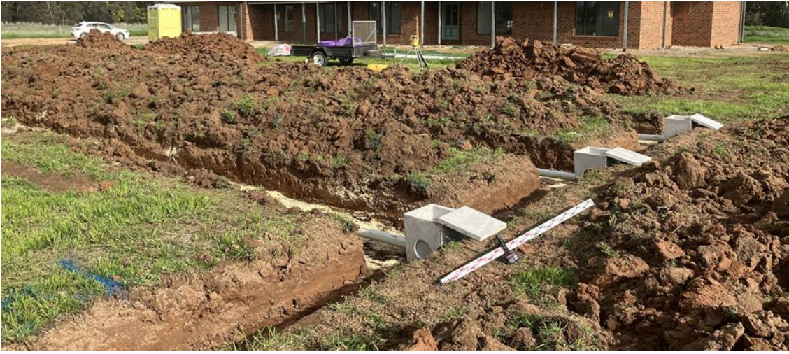
Image 14: An example of trenches laid in a series, spaced 2m apart.
