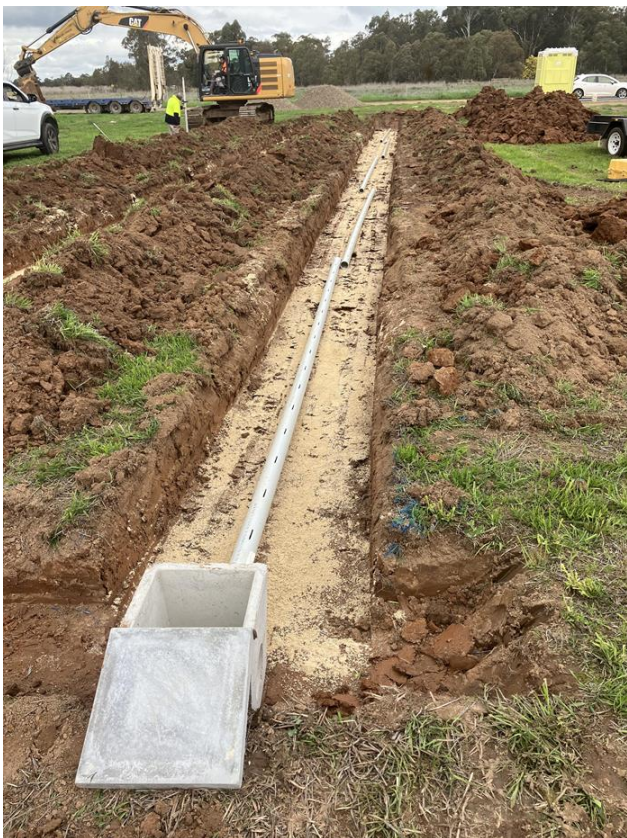
Image 11: Evapotranspiration trench with gypsum sprinkled along the bottom of the trench. Trench is 400mm deep and 1m wide
