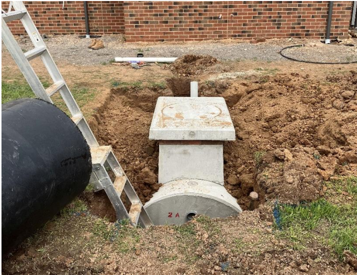
Image 8: Only the lid of the septic tank and pumpwell with alarm are visible when backfilled.
