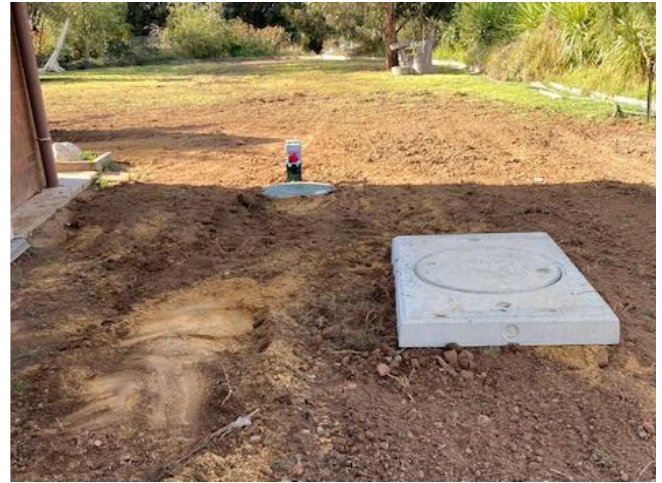
Image 8: Only the lid of the septic tank and pumpwell with alarm are visible when backfilled.
