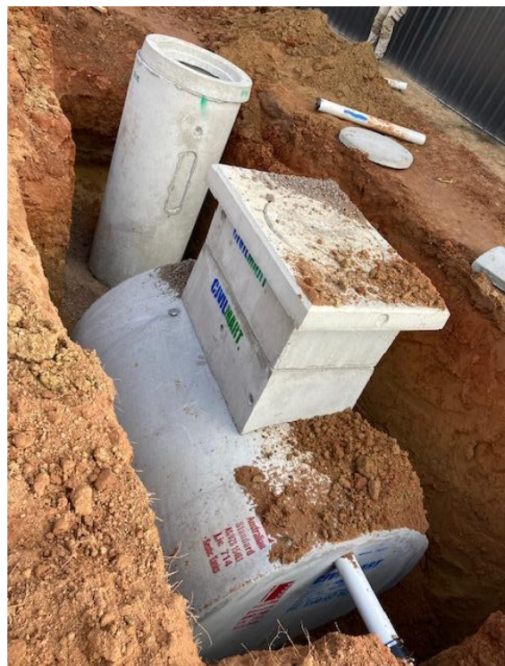
Image 7 – Septic tank with riser lids finished at ground level. All waste septic tank with risers extended to ground level to ensure access for pump out and other maintenance. Pump well installed at the outlet of the septic tank to pump to effluent disposal trenches.
